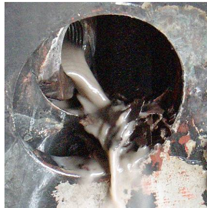
Scale washed out of FCAF N o .3. The scale shown was all removed by chemical action. No mechanical action was required. © M.Bane
